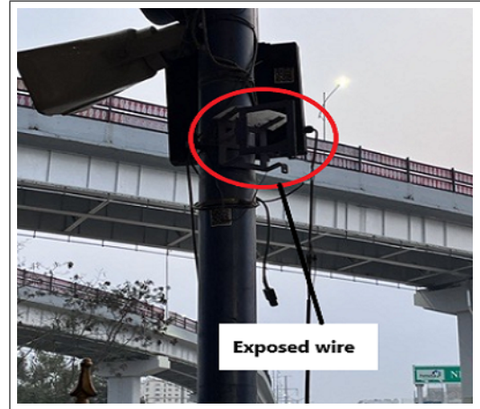
(b) After stealing the device wire is exposed which can be dangerous
