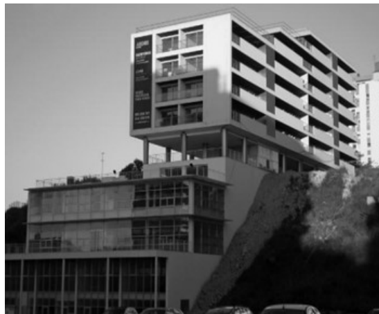
Fig. 2.9: Mass irregularity in vertical direction
