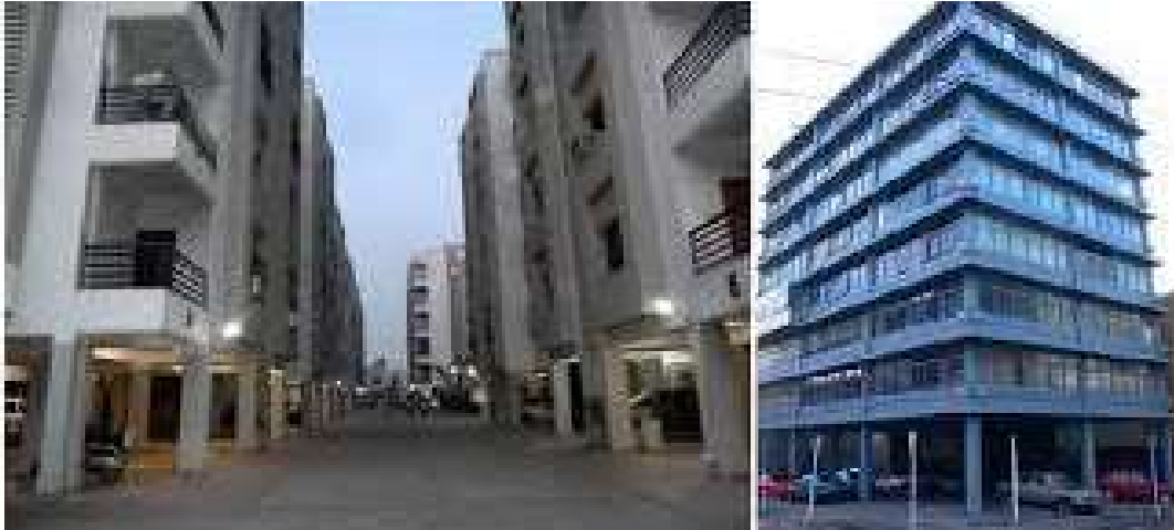
Fig. 2.6: Buildings with soft storey
