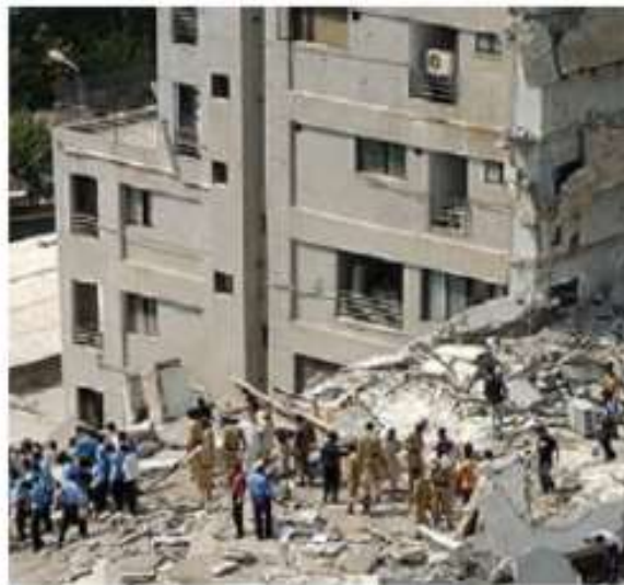
Fig. 2.7: Building with setback irregularity.
