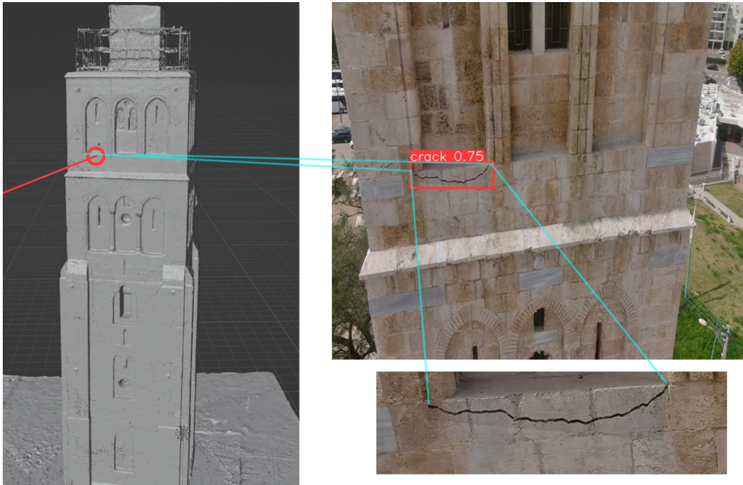
Figure 5.4 3D mesh model of the building (left) with marked crack using 2D to 3D mapping shown using the red ray and red ring; Captured image of the building (top-right) using UAV showing the crack predicted using YOLOv5 [1]; Zoomed-in Crack (bottom-right); Correspondences of all the three images are shown using blue lines.
