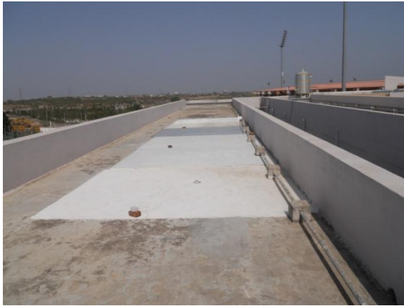
Figure 3.1: Cool roof installed on site
