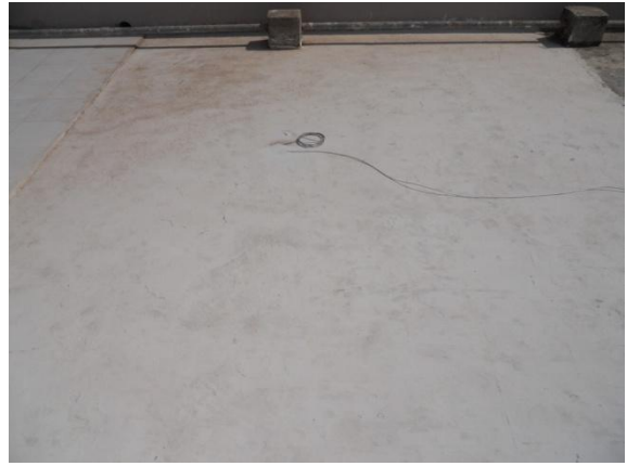
Figure 3.2: Cool roof installed on site
