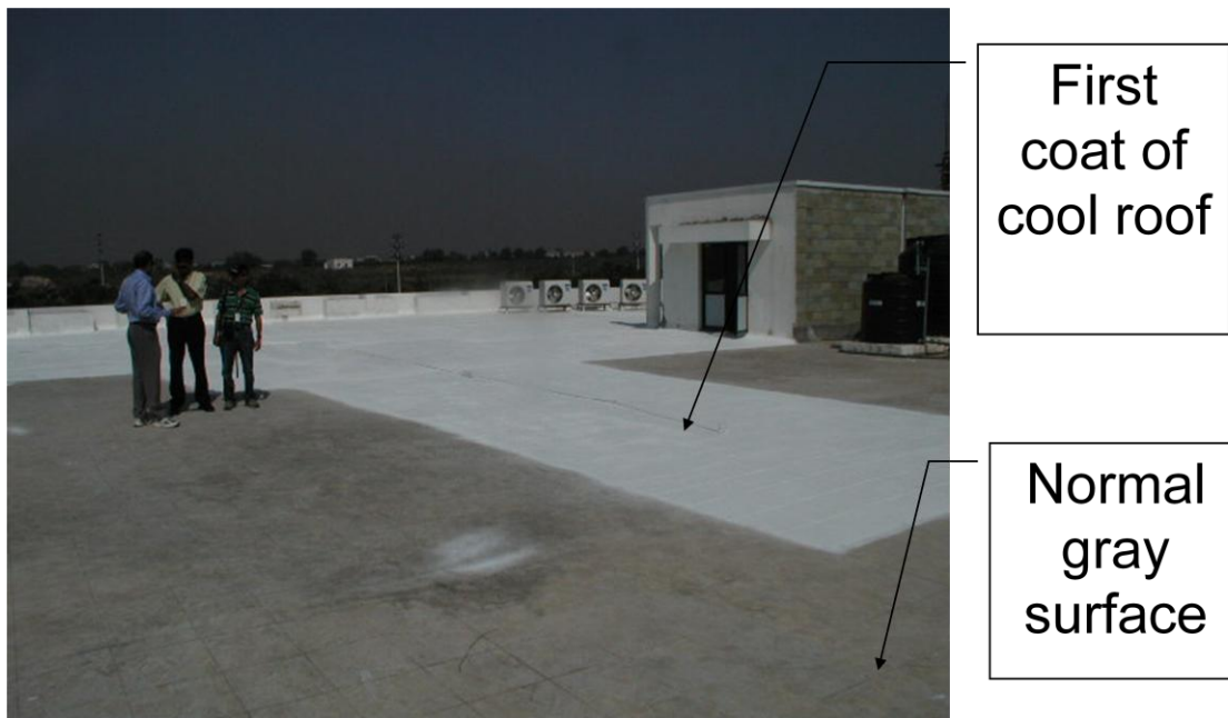
Figure 4.5: Coating work under process at the field experiment site
