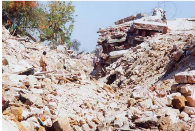
Fig. 2 Extensive damage occurred in non-engineered structures
