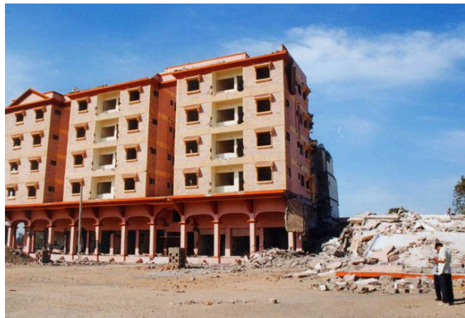
Fig. 3 Soft bottom storey
